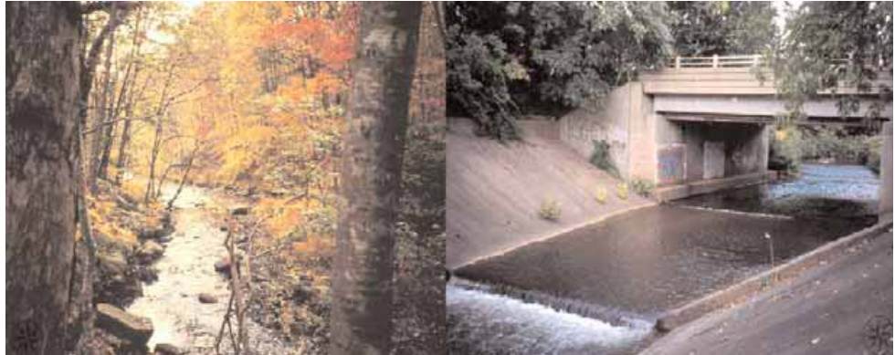
Figure 2. Changes in stream form associated with urbanization.
